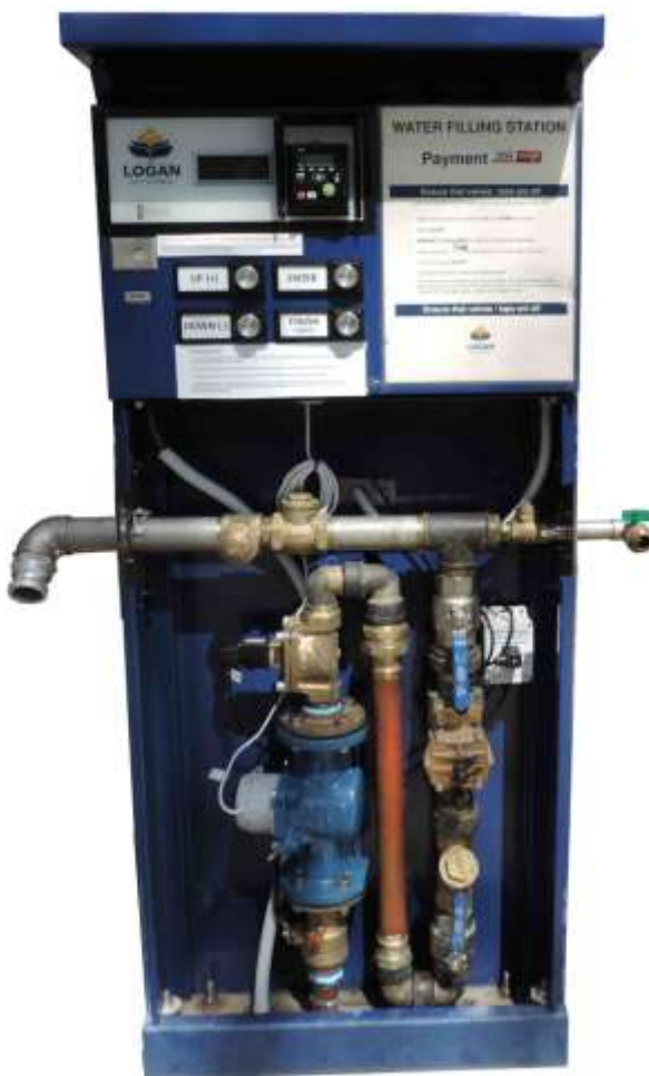
Figure 3 - WD2500 with internal backflow prevention
