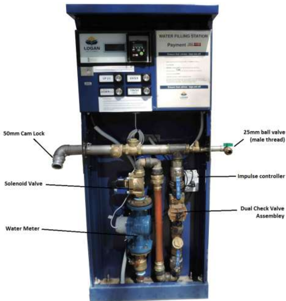
Figure 7 - WD2500 with internal backflow prevention
